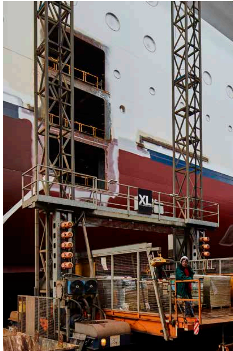
Application of surface protection
