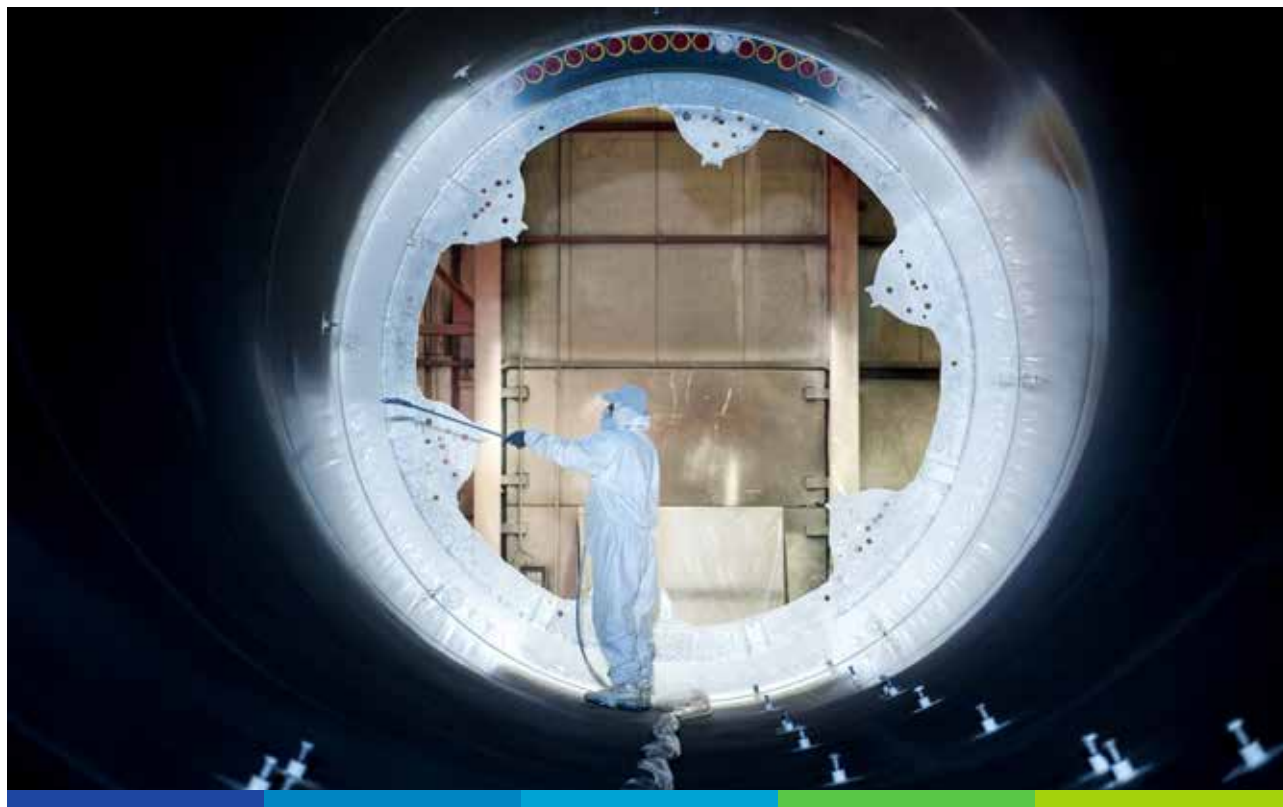
Surface protection work on a wind turbine
