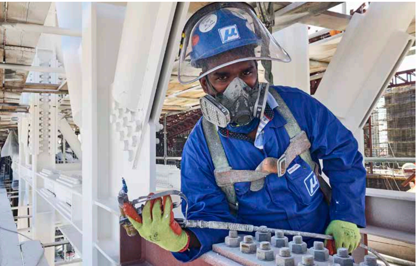
Application of passive fire protection
