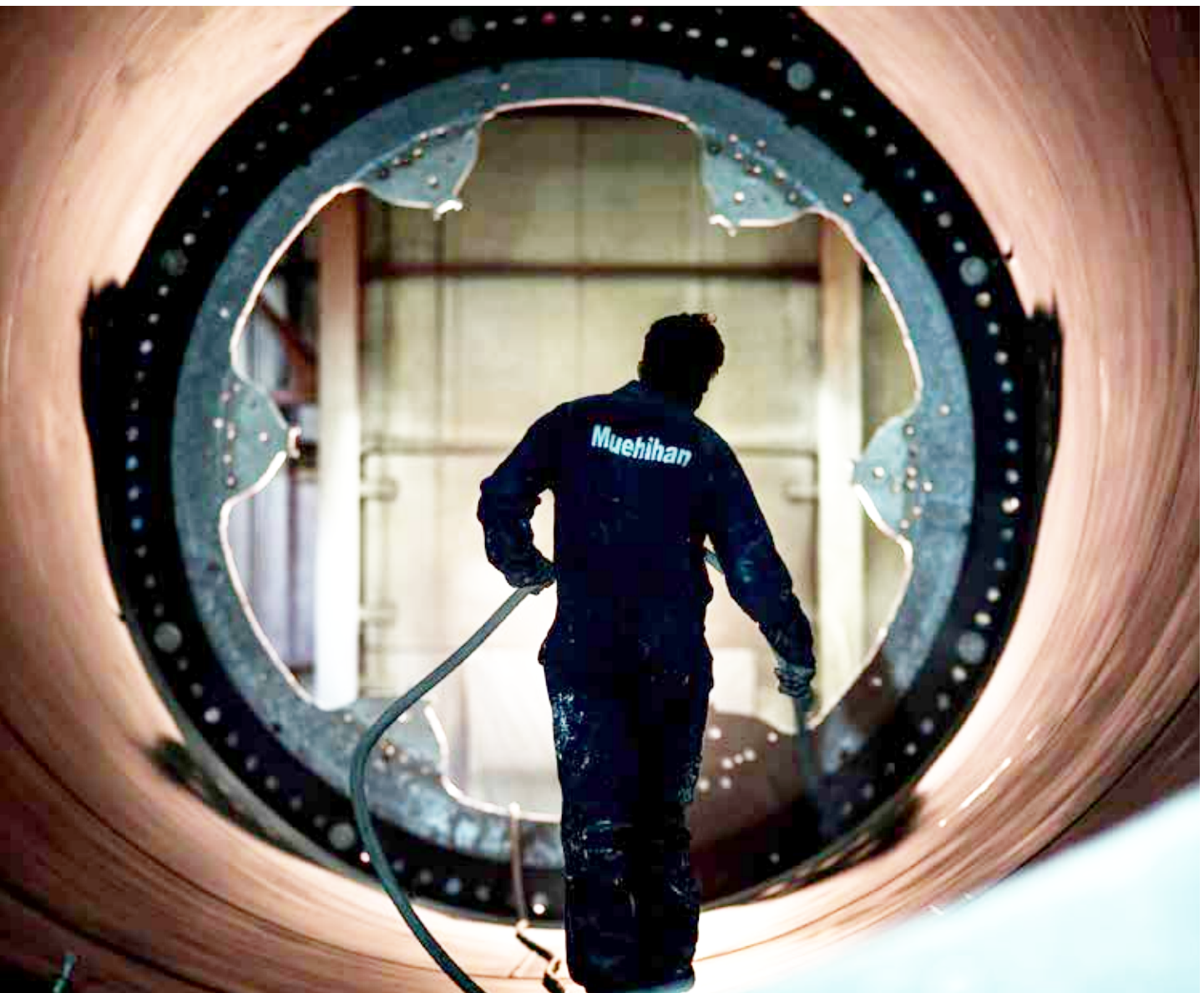
Preparations for application of surface protection on a wind turbine
