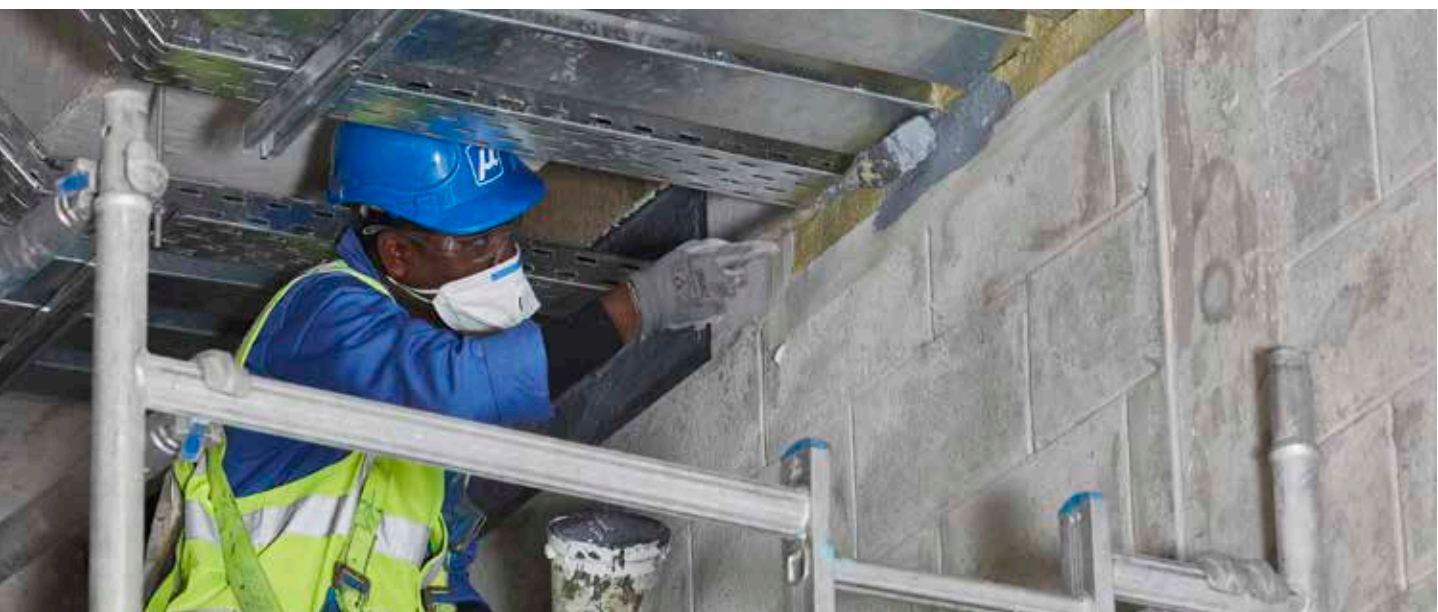
Application of passive fire protection
