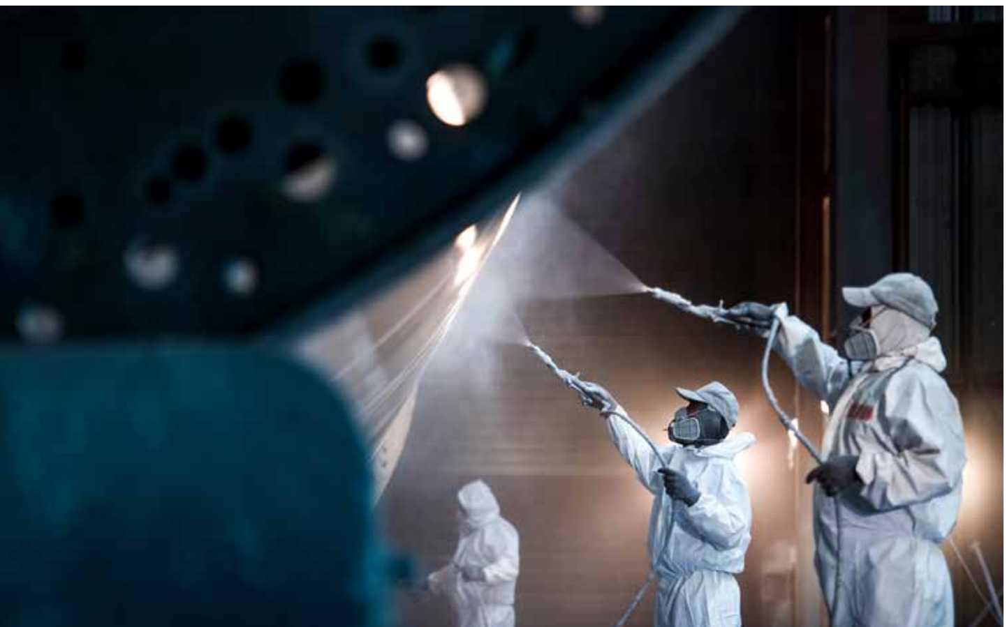
Application of surface protection on a ship's hull
