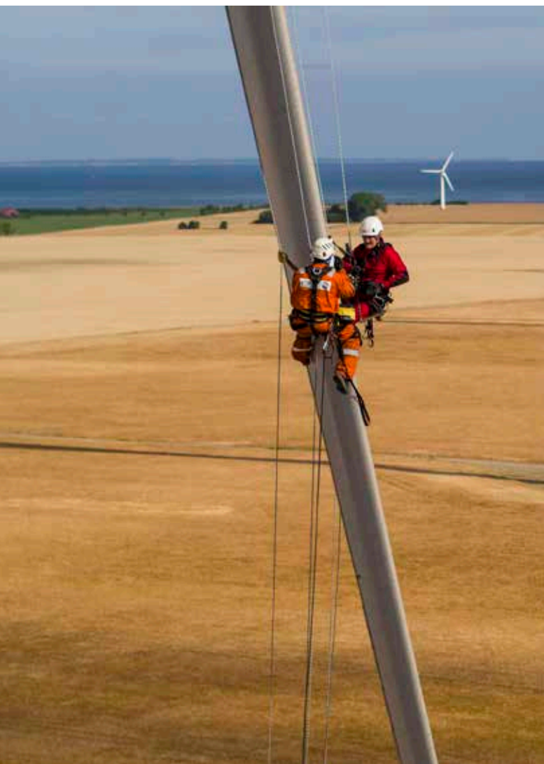
Inspection of rotor blades on wind power stations
