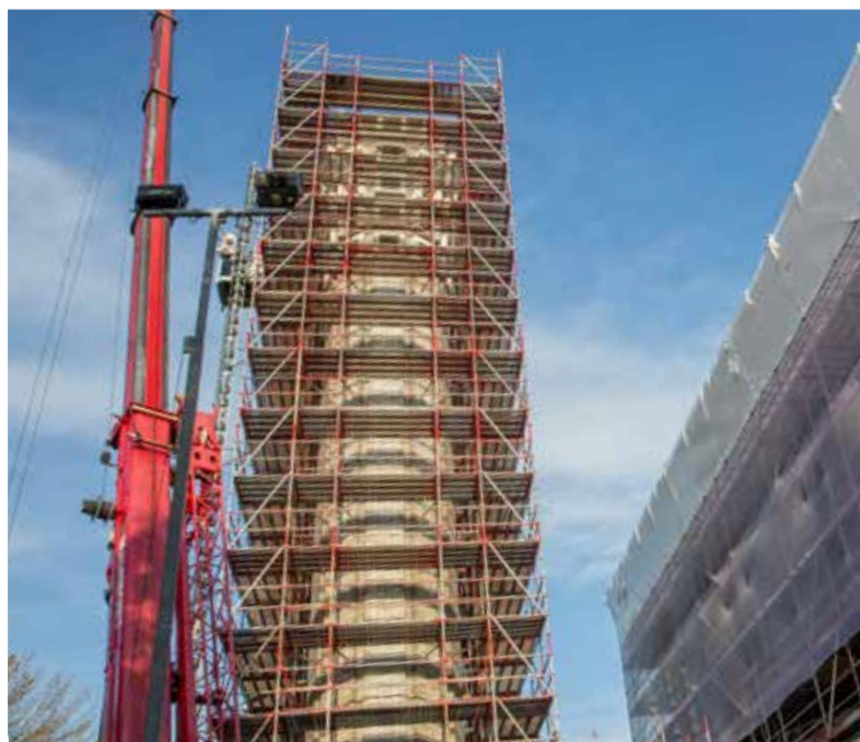
Scaffolding work on an industrial plant
