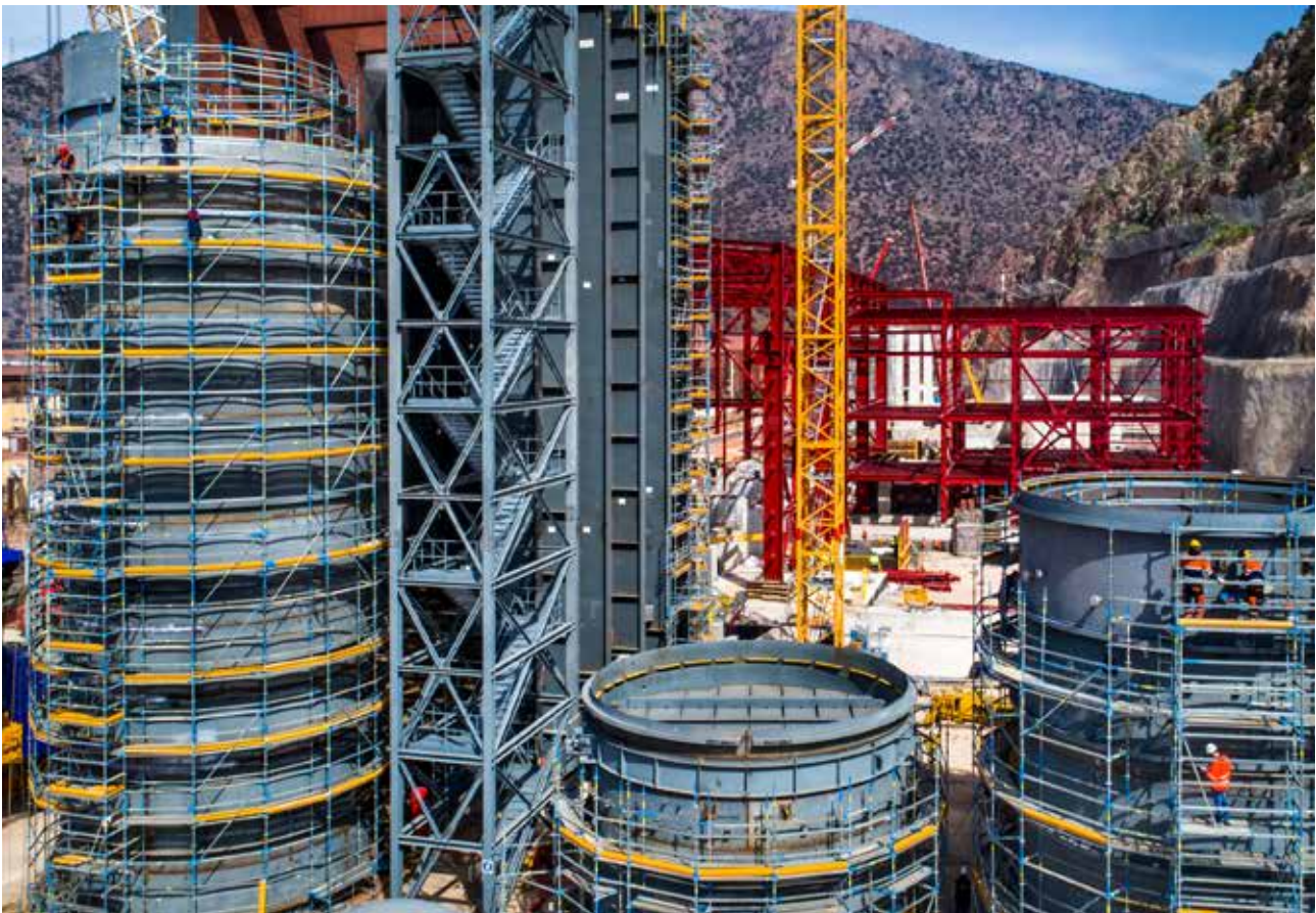
Scaffolding work on an industrial plant
